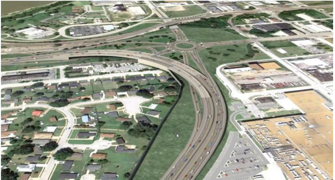
Upgrades to Interstate 55 Downtown will include the construction of a new roundabout, located at the current Crump interchange. (Screen grab)
