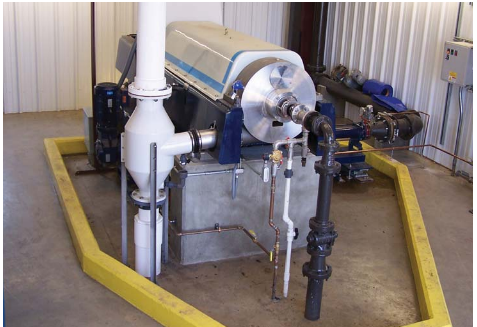
Above: The demolition of several sand drying beds allowed utilization of available space and allowed existing sludge lines, water lines and drains to pipe supernate back into the plant. Below: The Andritz D5L, has a throughput of 1400 pounds per hour or 100 gpm at the current 3.3 percent solids.
